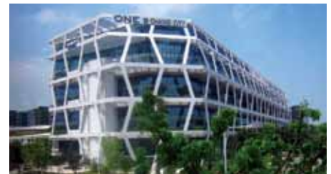
ONE@Changi City Integrated business park space complemented by retail mall and hotel, Singapore
